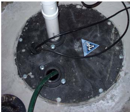
(Insert hose into access hole.)
