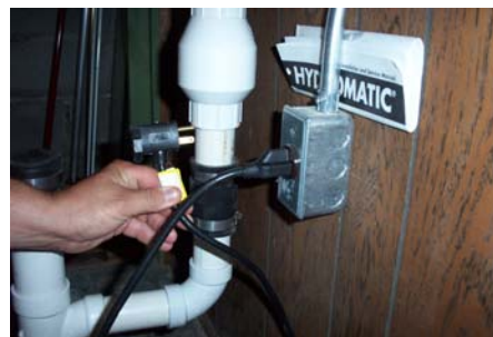
(Pump motor cord directly to outlet.)
