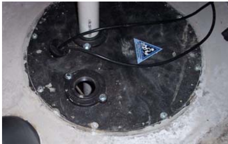
(Access hole in lower-left corner.)
