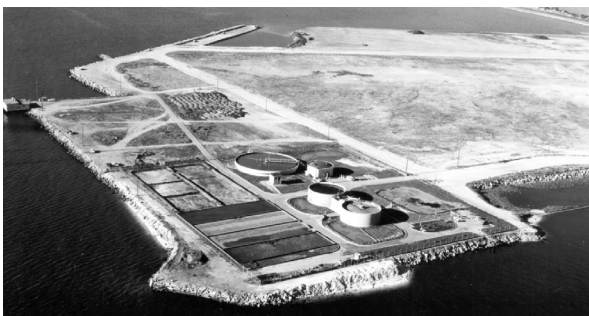
The Stege Sanitary District’s Point Isabel primary wastewater treatment plant opened in 1955.
