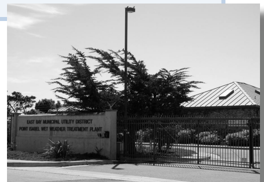
Today, East Bay MUD operates a wet weather wastewater treatment plant at Point Isabel.
