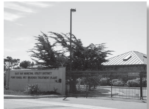
Point Isabel wet weather wastewater treatment plant
