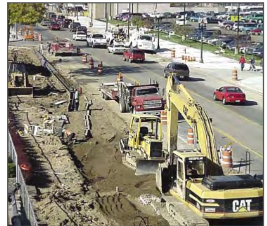
Michigan Avenue Sewer Separation Construction
