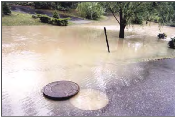
Surface Flooding and Sanitary Sewer Overflow
