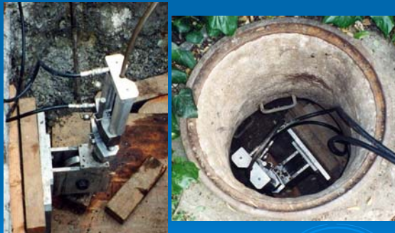
HDPE Installation Small Machine in Pulling Pit/Manhole
